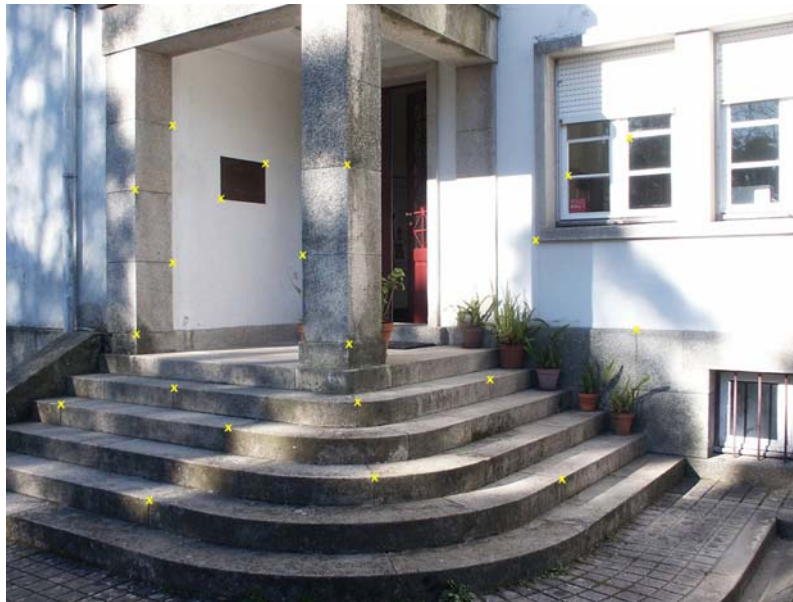
Figure 4: Façade with known absolute coordinates used in orientation procedure.
